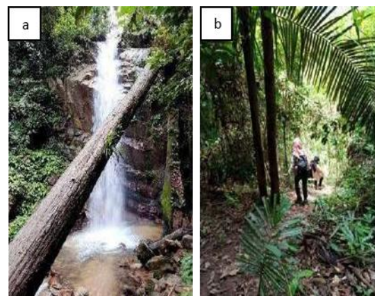
Figure 7. a) Actual risk of fallen trees at Batang Taye Waterfall; b) Potential risk of landslides due to the steep cliffs.
