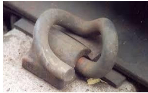
Figure 10. An Example of a Pandrol Fastening
